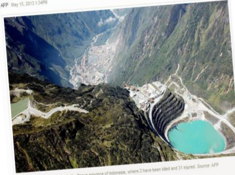
The Freeport Grasberg mine in the Papua province of Indonesia, where 2 have been killed and 31 injured. Source: AFP RESCUERS have recovered four bodies and rescued 10 of the dozens trapped underground after a tunnel caved in at a giant US-owned gold and copper mine in eastern Indonesia.
