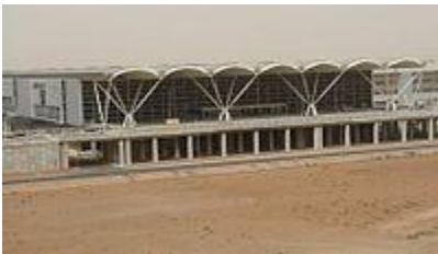
Front view of Erbil International Airport under construction in 2008
